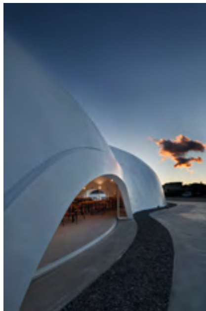
Takeshi HOSAKA, Restaurant Hoto Fudo , Fujikawaguchiko, 2009 © Takeshi HOSAKA Architects © Nacasa & Partners Inc. / Koji Fujii
